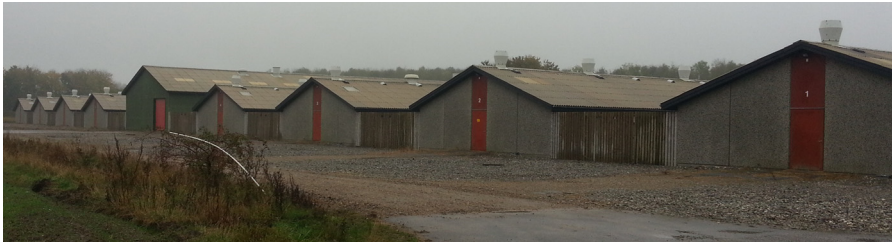
Fig. 2. The wooden walls separating shielding the space between the sections. The photo is taken on the East-side of the station.
