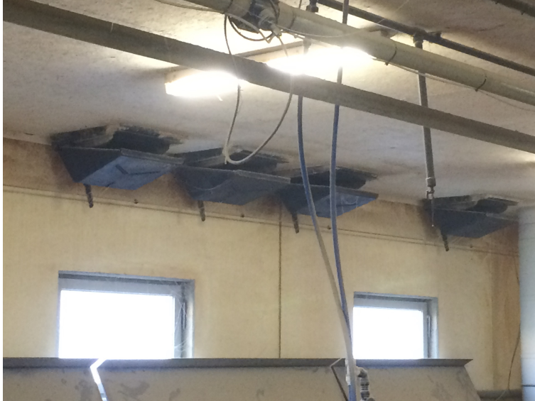
Figure 1.9: Ceiling inlets in the weaner section.
