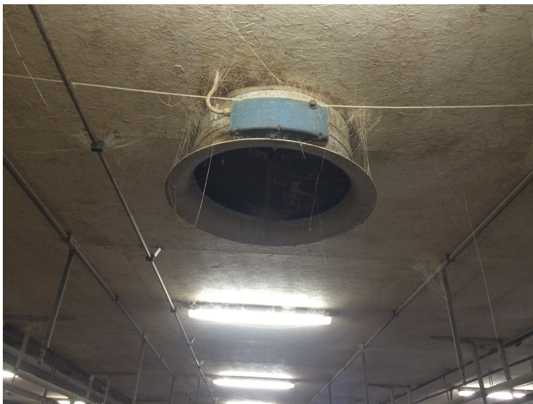
Figure 1.10: Exhaust fan in the weaner section.
