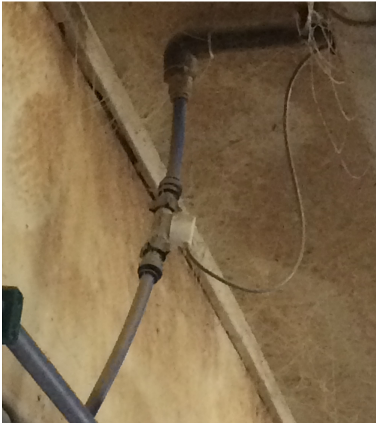
Figure 2.7: Water flow meter installed on the water pipe of a water cup.
