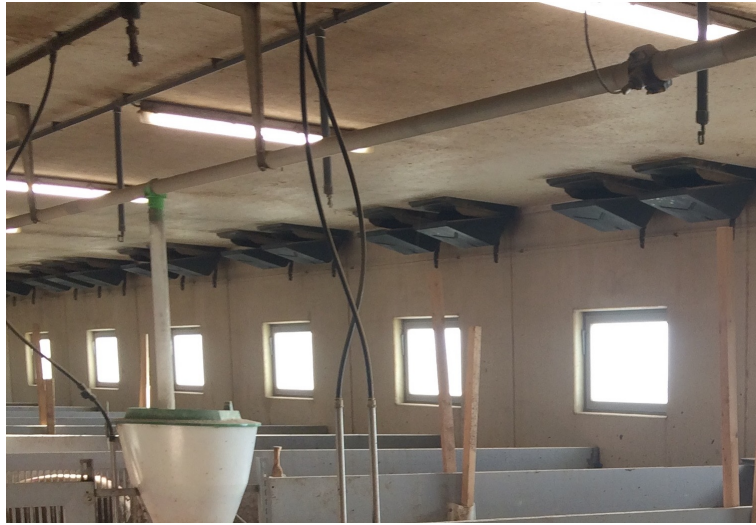
Figure 1.11: Ceiling inlets in the finishing section.
