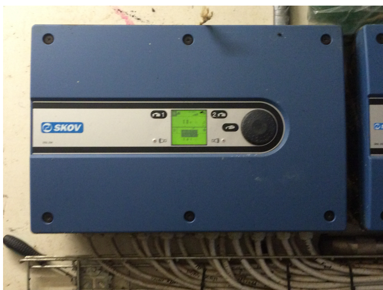
Figure 1.7: Dol 234 two-section-control climate computer from Skov A/S.
